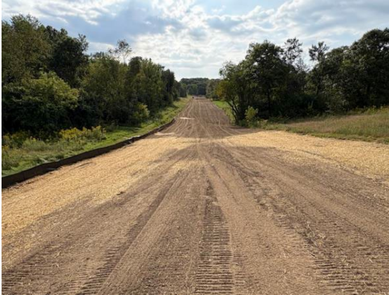
Facing west near MP 2.8; upland area topsoil and seeding complete, mulching in progress
